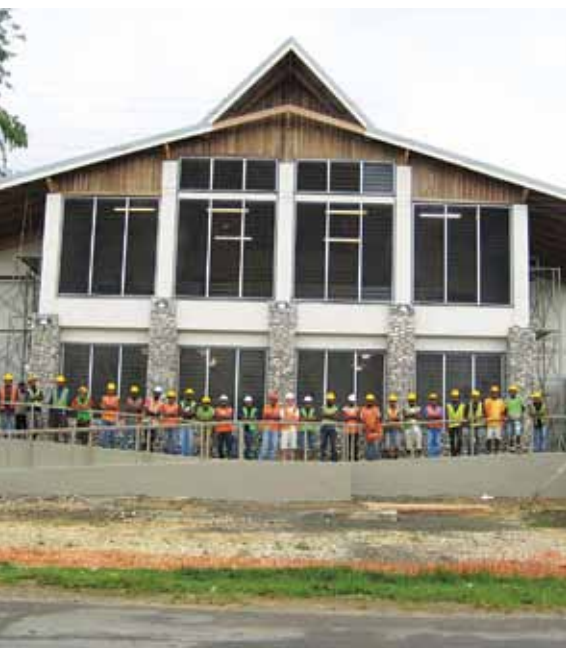
With RAMSI's assistance, much of Solomon Islands' justice infrastructure—such as the Malaita Magistrates Court—has been rebuilt.
